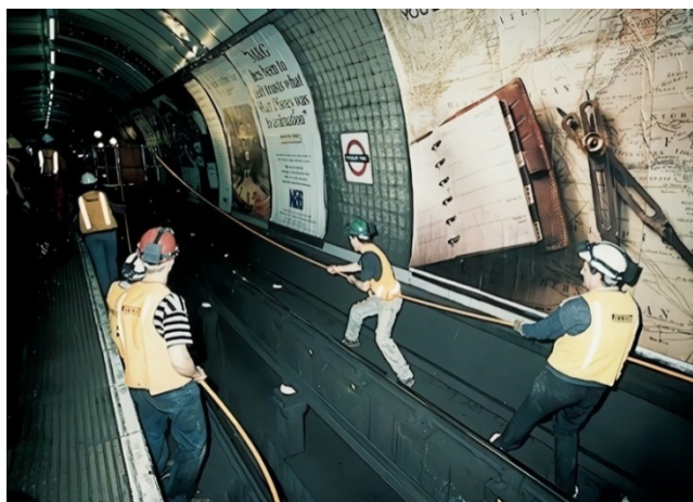
Figure 4. Installation of optical cable through a metro system (source: FTTH Council)
